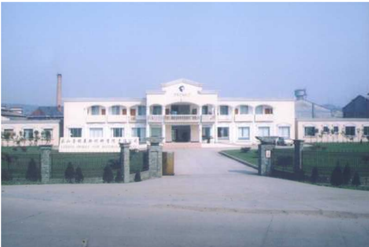
Administration Block & Factory, Primet, Sichuan, China
